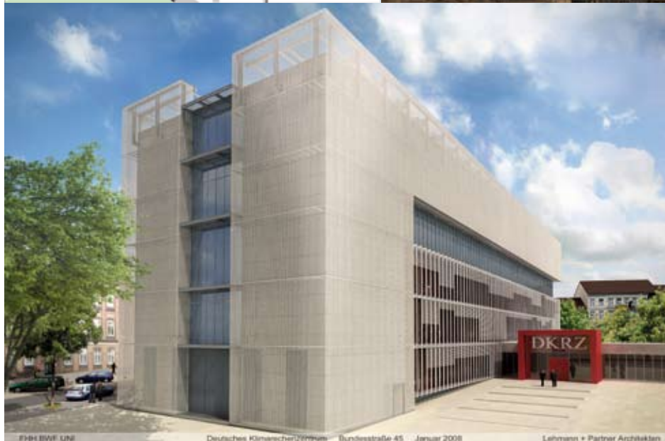
Figure 1: At the end of 2008 DKRZ will move into a new building. View from the Bundesstraße to the projected DKRZ building which will not only accommodate the new supercomputer HLRE II but also the offices of DKRZ and M&D employees. Top left: Map showing the location of the new DKRZ building. Top right: Construction site – the existing building will be fundamentally reconstructed.
